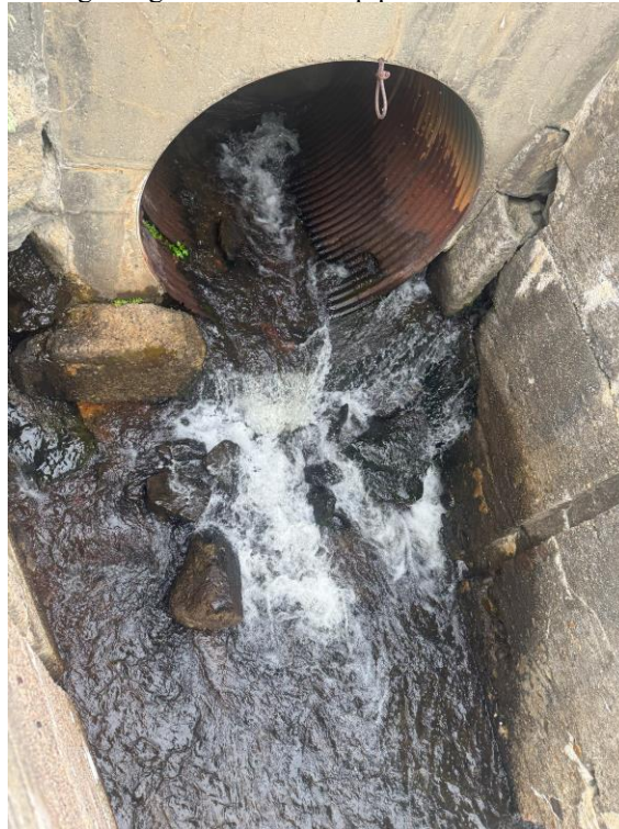
Photo 2. 6-foot diameter corrugated galvanized metal pipe on downstream side of sluiceway structure
